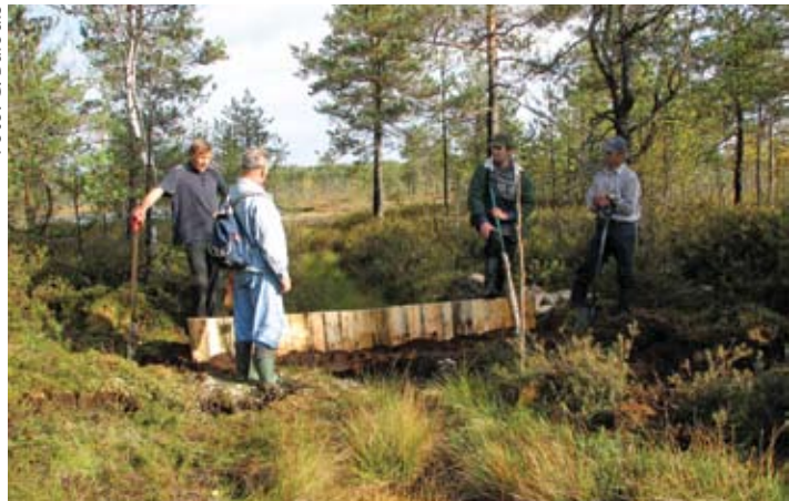
Kombinētā kūdras-koka aizsprosta būvniecība Cenas tīrelī. In Cena Mire there are build dams by hand that consist from peat and wooden planks.
