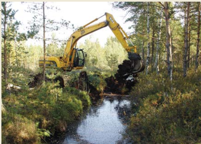
Dambja būve ar ekskavatoru 22.09.2006. Building of peat dams by excavator, September 22, 2006.
