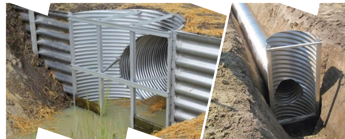
Figure 1. Controlled drainage sample in a ditch [16]
