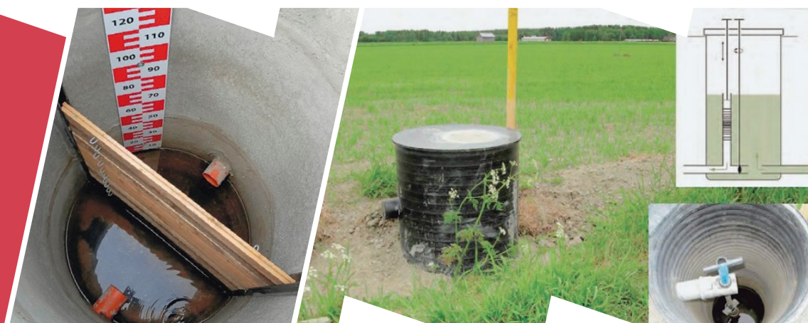
Figure 5. Adjustable gate system with wooden boards in the drainage control well. Photo: R. Abaja
