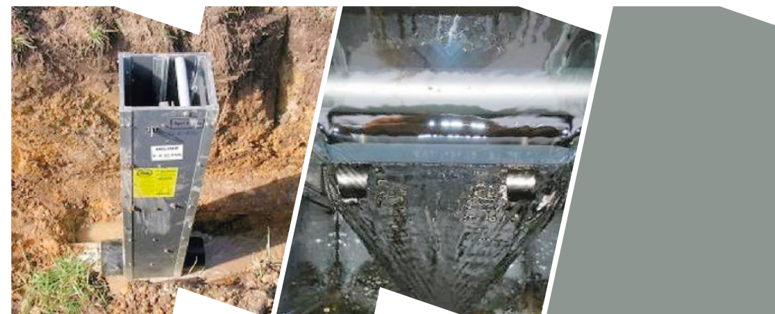
Figure 4. Stainless steel control well with gate for regulating water run-off from the field with a covered drainage system installed on the drainage collector. Figure on the left – drainage control well. Figure to the right – internal view of the well at the water overflow over a gate set at a certain height [16]
