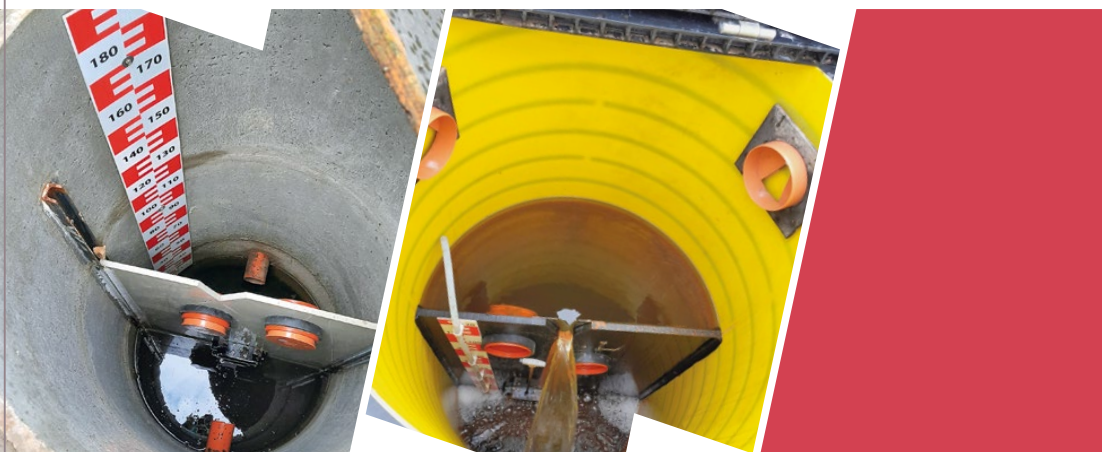
Figure 2. Reinforced concrete framework control well with gate construction for regulating water run-off from the field with covered drainage system. An example of a drainage control well built in the LIFE CRAFT project in the Menģele pilot area. Photo: R. Abaja
